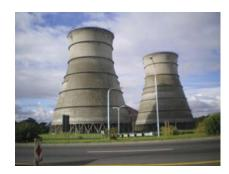
FIGURE 14–32 Two natural draft cooling towers on a roadside. ©Yunus Cengel
