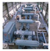
FIGURE 7–70 A large compressor assembly. Photo courtesy of the Dresser-Rand business, part of Siemens Power & Gas
